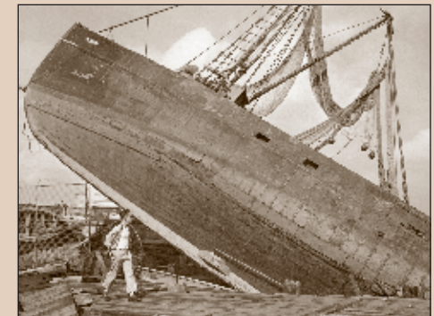
Hurricane Carol strikes Port of New Bedford, 1954.
