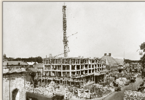
New Bedford Hotel under construction, 1918.
